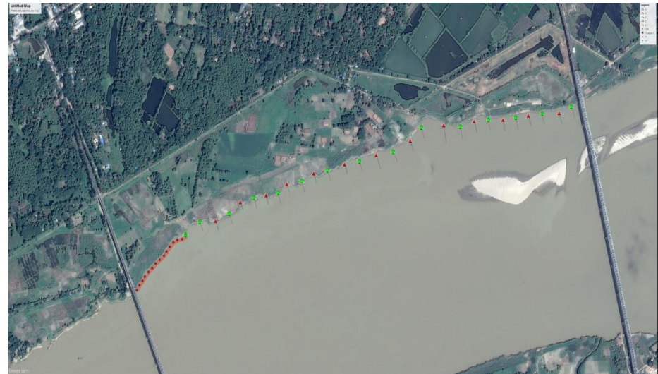
BANK PROTECTION STRUCTURES IN UPSTREAM OF THE BOMYATHUN BRIDGE
