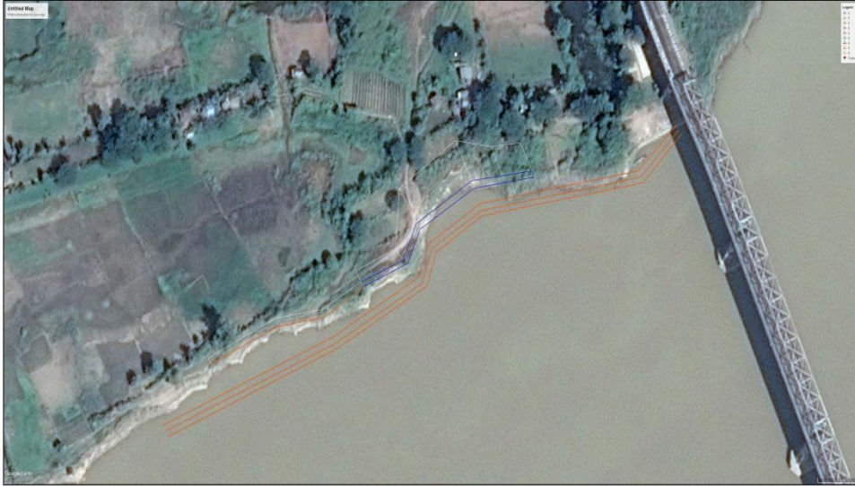
BANK PROTECTION STRUCTURES AT DOWNSTREAMS OF BOMYATHUN BRIDGE
